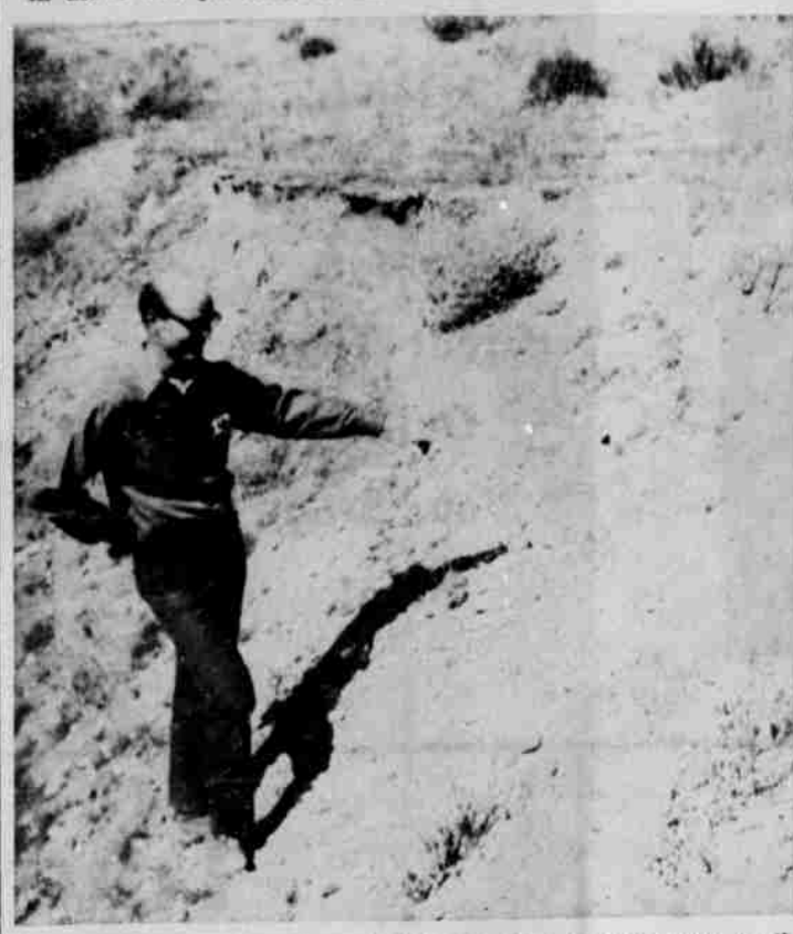
ALTHOUGH THE bank has sluffed off, Dale Boner points to the gravel line that underlays Burbank soil down near Irrigon.
