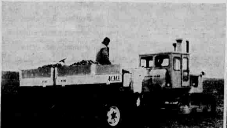
"OFF TO WORK WE GO" loaded and ready to plant. Dennis O'Donnell is on the planter and Omer Huston is driving cat.
