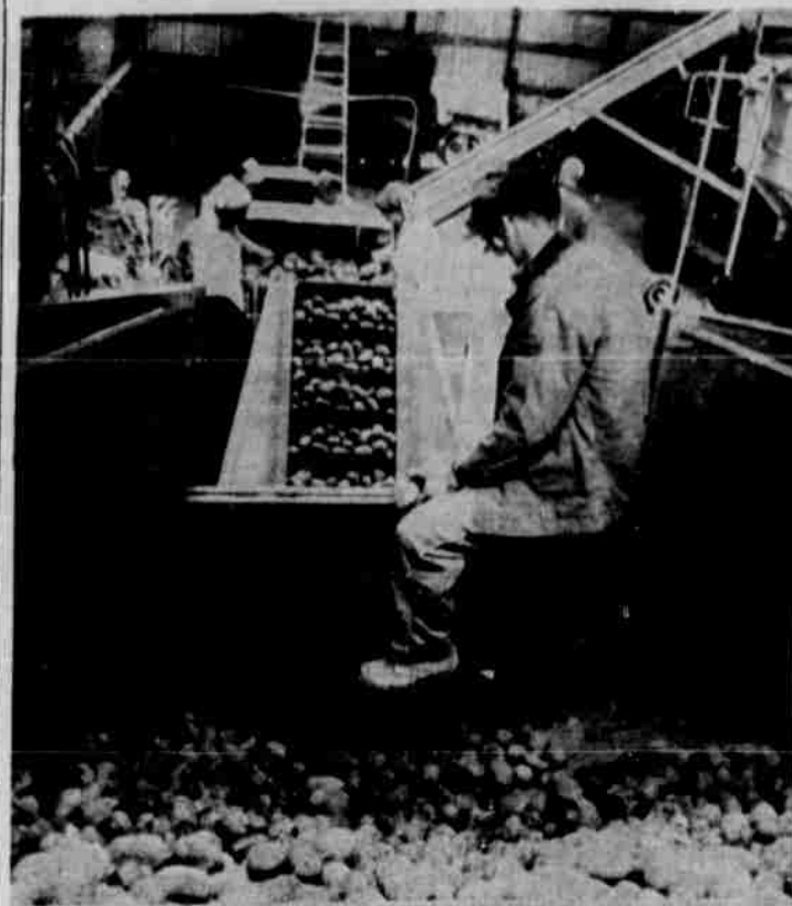
POTATOES HAVE their ups and downs these days at the D. O. Nelson ranch. Steve Rea keeps an eye on them as they are going down through a hole in this specially built truck into a bin to be picked up on the conveyor belt seen in the center of the picture. Up they go to be sorted on specially built rollers where they are cut according to size.
