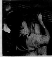
hidden in the ceiling. Furniture can be placed anywhere because floor or wall space isn't needed for the heating units. Ceiling cables are stapled to plaster laths or dryboard and then covered by plaster or dryboard. The heat radiates down... just like the sun shining from above.
