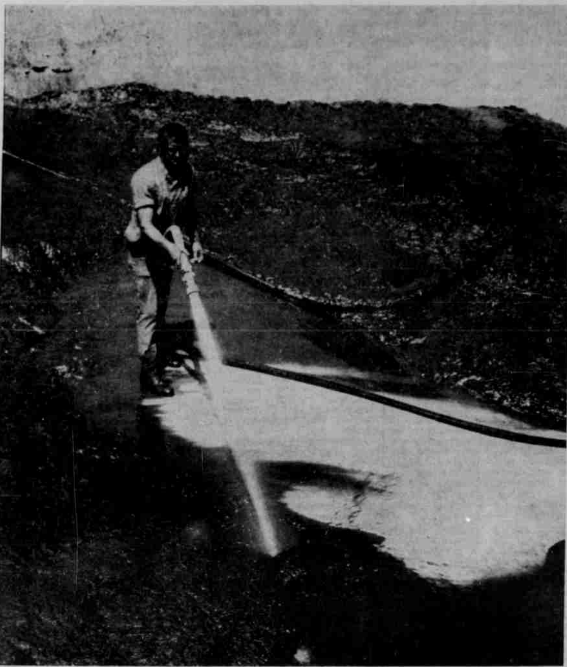
ALL ALONE IN A SEA OF MUD is Wayne Harsin, City of Heppner employee, as he washes down the city's swimming pool early this week. The city crew washed seven feet of mud, a result of last week's flood waters, out of the pool by using fire hoses. As of Tuesday, the pool was refilled and workmen were cleaning the deck and poolhouse. (G-T Photo).
