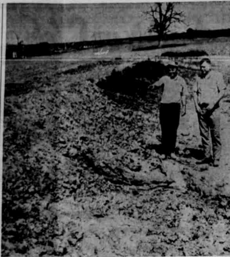
RUDY BERGSTROM (left) shows dam of watering pond to County Agent Harold Kerr. Bergstrom built the dam last year but heavy runoff water from snow melt cut through it this spring. Repairs will be made. (G-T Photo).
