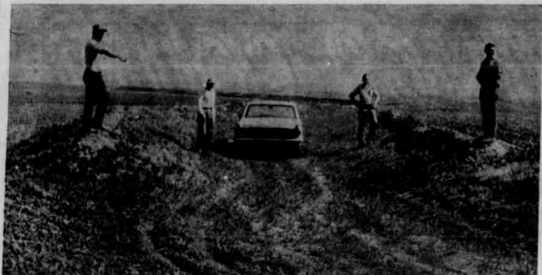
RUDY BERGSTROM, 1969 Conservation Man, points out how he solved a water runoff problem on his place. He stands at left on the end of an embankment that prevents water running down slope to the left, but the contour changes here, and the embankment at the right, which continues on out of the picture, keeps the water from running down the slope that now veers to the right. Jack Sumner, chairman of the selection committee, stands at right. Bill Bergstrom, Rudy's father, stands by car (left), and County Agent Harold Kerr is at the right of the car. (G-T Photo).
