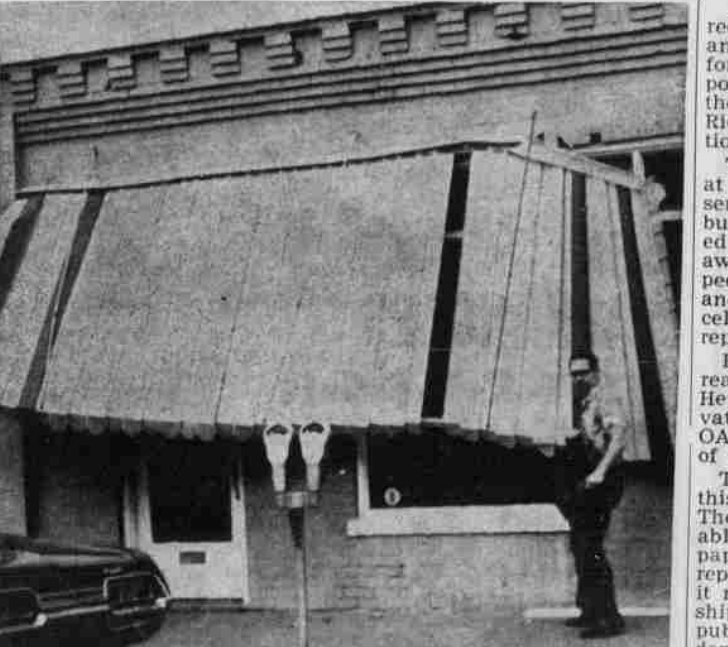
STRONG WINDS whipped through the Heppner area Tuesday, reminiscent of the Willamette Valley's Columbus Day storm of a few years ago. One gust caught the metal awning at the Gazette-Times office and ripped it loose, threatening—but failing—to smash a big plate glass window in the process. Foreman Arnold Raymond helped secure the awning to keep it from causing more damage. (G-T Photo).
