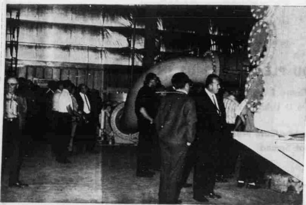
TO TELL AN ACCURATE story, this picture should have another dimension, that of sound. Noise in the building that houses the turbine and compressor of Pacific Gas Transmission Company at its Ione installation was so great that Lions and Chamber members visiting there September 23 couldn't speak above it. Lions President Herb Ekstrom, Jr. (right) peers through a glass peephole to watch combustion in the gas-fueled turbine. (G-T Photo).
