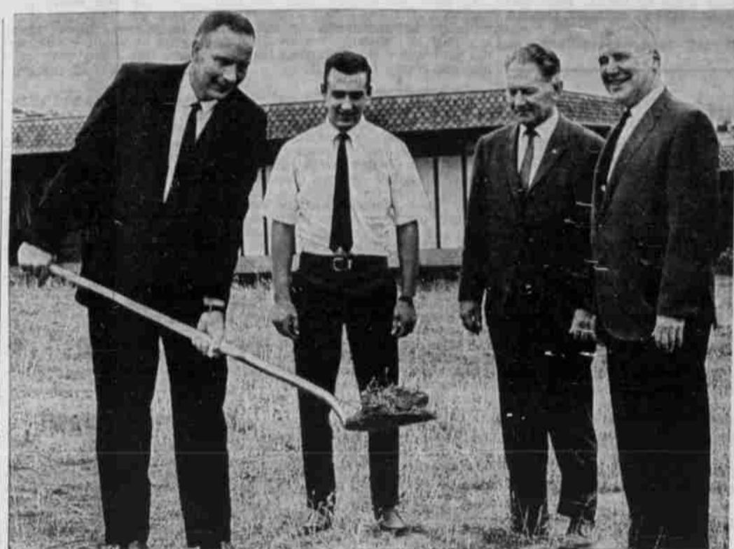
ROBERT ABRAMS, chairman of the board of directors of Blue Mountain Community College, takes first shovelful of dirt in breaking ground for the third BMCC building in Pendleton. Taking part with him are Tom Rugg, Pilot Rock, student body president; Ford Green of Jensen-Green, Inc., general contractor; and President Wallace McCrae of the college.
