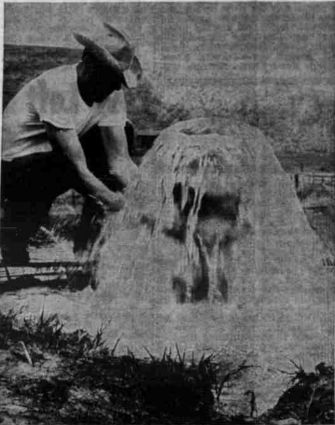
HAPPY is the rancher who brings in an artesian well! (Even happier than one who gets an inch or so of rain at a critical time). Such an extra-happy rancher is Don Evans who is shown Saturday working at capping the new well on the ranch owned by himself and his mother, Mrs. Millie Evans, between Heppner and Lexington. The well, 250 feet deep, is figured to be flowing at the rate of some 800 gallons per minute and, with pumping, would produce considerably more water. Hidden by the flow of water here is the valve that Don is applying. (See other photos on page 6).
