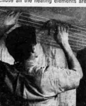
and then covered by plaster or dryboard. The heat radiates down... just like the sun shining from above. Thermostats control the temperature in each room so you always have the most comfortable degree of warmth. Ceiling cable is safe, clean and the most convenient way to heat
