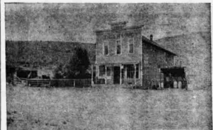
THIS IS HOW the Cecil store and post office looked in 1914 after Thos. H. Lowe bought it and made repairs, giving it new paint and making other improvements.
