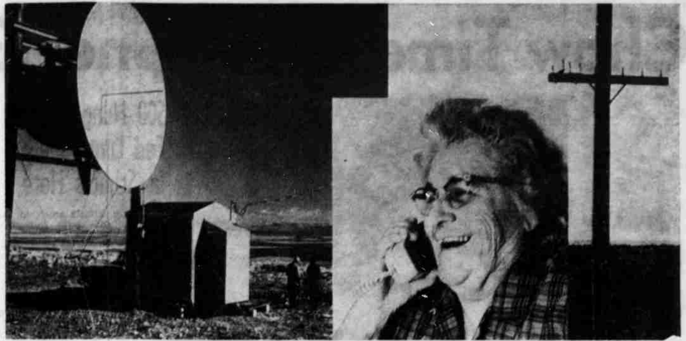
HAPPY SMILES like Elsie Bennett's of Crane, (inset) were familiar sights in Harney county March 18 as residents in a 5,000 square mile area of the county began enjoying phone service for the first time. Pacific Northwest Bell built a central office, installed phones, erected microwave towers (left) and strung
