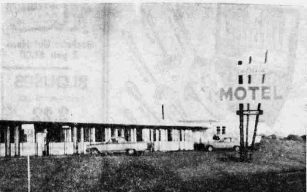
ONE OF TWO fine motels already open to the public at Boardman in its new location is the Riverview Motel. Eventually, the three motels will have 100 rooms to furnish accommodations. The town will be able to handle small conventions.
