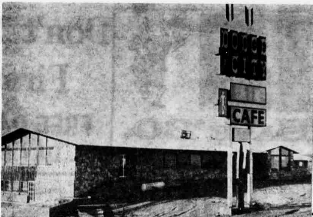
NOW UNDER CONSTRUCTION is Joe Tatone's Dodge City, which will be an ultra-modern restaurant motel. The facilities will accommodate up to 300 in the restaurant, which is shown here. The motel section, yet to be constructed, will be located out of the picture at the right.
