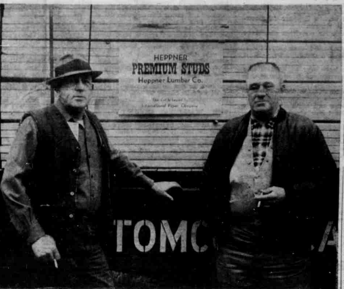
BARNEY MALCOM (left), owner of Heppner Lumber Co., and Ed Brandenburg, sales manager, stand beside load of premium studs on the new-style Tomco freight car. (G-T Photo).
