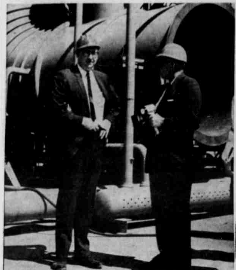
DON'T LET THE hard hats fool you! These aren't Boeing officials nor technicians—just Wes Sherman, editor of the Heppner Gazette-Times, and George Lindsey of The Dalles Chronicle standing near the base of the huge saxophone-shaped diffuser pipe at the Boeing test stand on the Boardman site. The pipe is designed to dissipate blast from rocket engines above. (Photo by Dean Holmes, Hermiston Herald).
