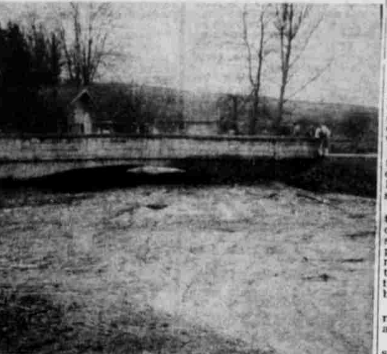
THE GALE STREET bridge had just about all it could handle last Thursday when Hinton Creek flooded. This picture is taken at the confluence of Willow Creek (coming in from left) and Hinton (at right). A little light is still visible in the bridge aperture, but it couldn't have handled much more water. The new Main street bridges have been a boon in preventing flooding in this area. (G-T Photo)
