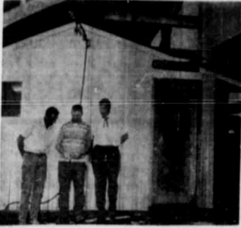
A NEW BUILDING , the rodeo office, has blossomed under the Buckeroo stands as one of several major improvements made to the fair and rodeo grounds this year. These three officials standing by the building look nonchalant, but actually they were quite apprehensive as the photo was taken. Sprinklers were dousing the area in preparation for the rodeo, and the three were threatened with drowning. From left are Director E. H. (Tod) Miller, Floyd Jones, rodeo chairman, and Jack Locke, rodeo secretary. (G-T Photo)
