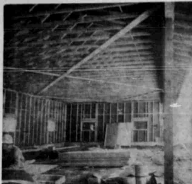
SPACIOUS INTERIOR of the large garage building at Tupper work center, now nearing completion, is shown in this picture. The structure will be large enough to shelter eight vehicles. (G-T Photo)
