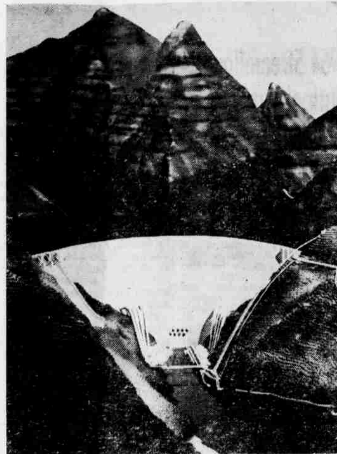
OUTPUT of hydroelectricity at massive High Mountain Sheep dam and powerhouse to be built on Snake River between Oregon and Idaho will be shared by Pacific Power & Light Company, one of four companies jointly sponsoring the $257-million multipurpose development. Its 58-mile-long reservoir will provide 3,600,000 acre feet of storage for flood control, recreational use and power generation. PP&L will get 279,000 kilowatts of initial output, later obtain 558,000 kilowatts of output when plant is doubled to 2-million kilowatts.
