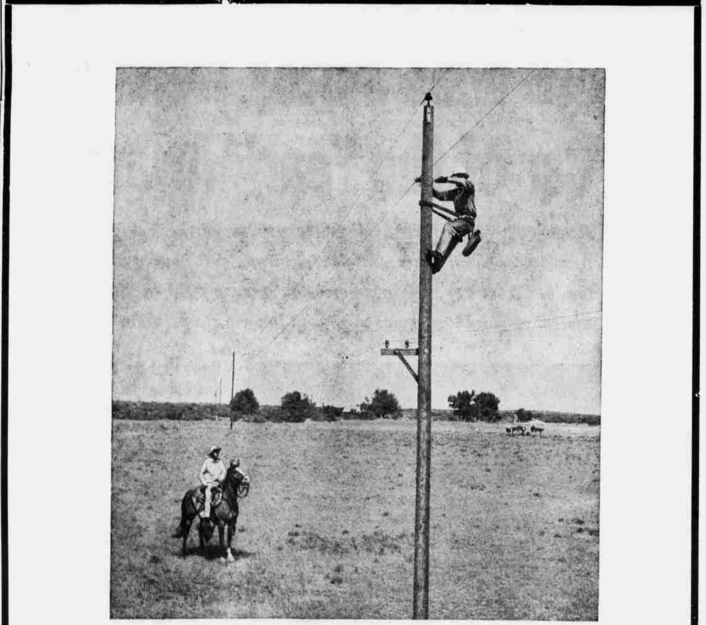
John McGuffin finally gets electricity in 1962, thanks to rural electrification
