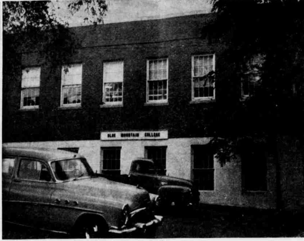
THIS BUILDING, located on South hill at Pendleton, houses much of Blue Mountain College at the present time. Automotive and other shop courses are held on lower level, and classrooms and offices are on second floor. The structure formerly was the Pendleton Technical school. Behind this building is John Murray Junior High school, which is shared between the college and junior high pupils, the college taking most of the second floor. A new site for the college has been purchased opposite the state hospital on the west side of town, following vote in the 2-county district, but building plans are held in abeyance now because of lack of funds. (G-T Photo)
