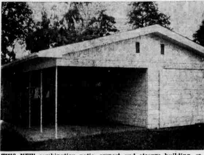
THIS NEW combination patio, carport and storage building, recently completed behind the Methodist church parsonage, largely by volunteer labor, is a part of improvements made on the church property during the past year. The church is entered in competition for the Sears and Roebuck Foundation church improvement award. (G-T Photo)
