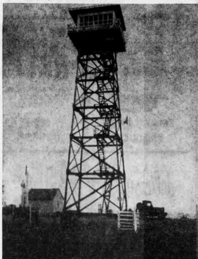
PROBABLY THE most comfortable of the three lookouts in the Heppner district of the Umatilla National Forest is the Wheeler Point lookout, which overlooks the John Day basin to the south. It was built in 1960, stands 67 feet high and has spacious 15x15 ft. quarters at the top. (G-T Photo)
