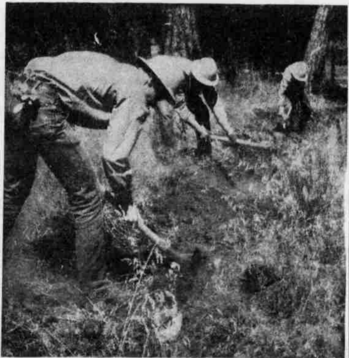
MEMBERS of the U. S. Forest Service fire suppression crew work in close cooperation in digging a fire trail with pulaskis and shovels. An 8-man crew, using three shovels and five pulaskis, can build about 1000 feet of 32-inch trail per hour. (G-T Photo)
