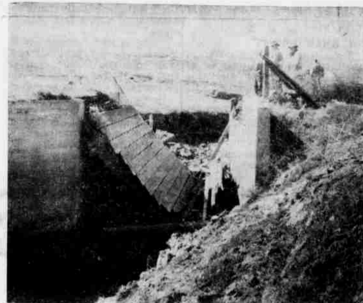
THIS WAS all that was left of a county road bridge in Blackhorse Canyon, three miles from Lexington, when a truck and trailer loaded with grain went through it Friday. The truck made it across but the trailer didn't. (G-T Photo)
