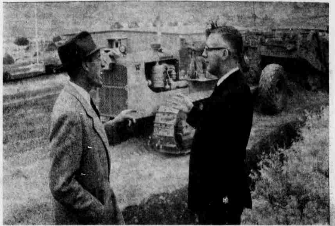
HEAVY CONSTRUCTION was underway Friday at the site of the new Heppner-Lexington High school when Dick Wilkinson (right), chairman of the board of directors of district R-1, and Superintendent Robert Van Houte went up to observe progress. Heavy equipment is shown working on excavation and the present Unit-A school, which will become a part of one wing of the new school, is in the background. The photo, taken in the rain, looks toward Heppner. (G-T Photo)
