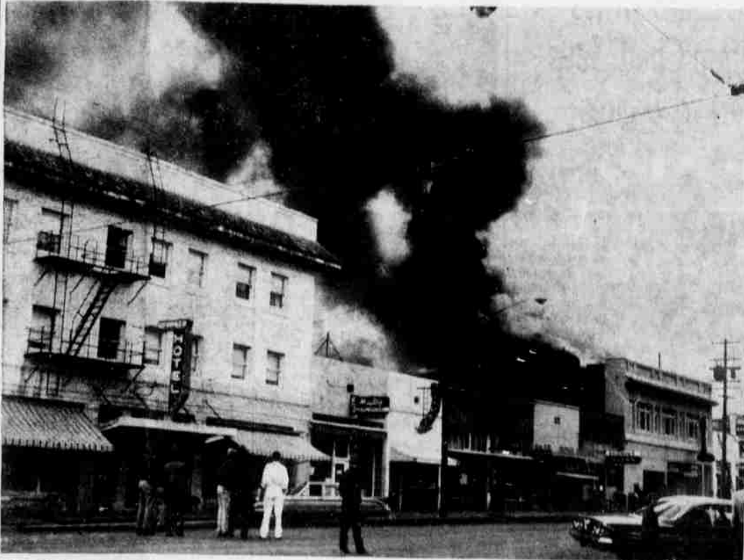
HERE'S HOW smoke was belching from the Elks' building shortly after the alarm was sounded Friday morning. Mrs. James McCabe spotted it from her home on the hill south of town and was first to turn in the alarm.
