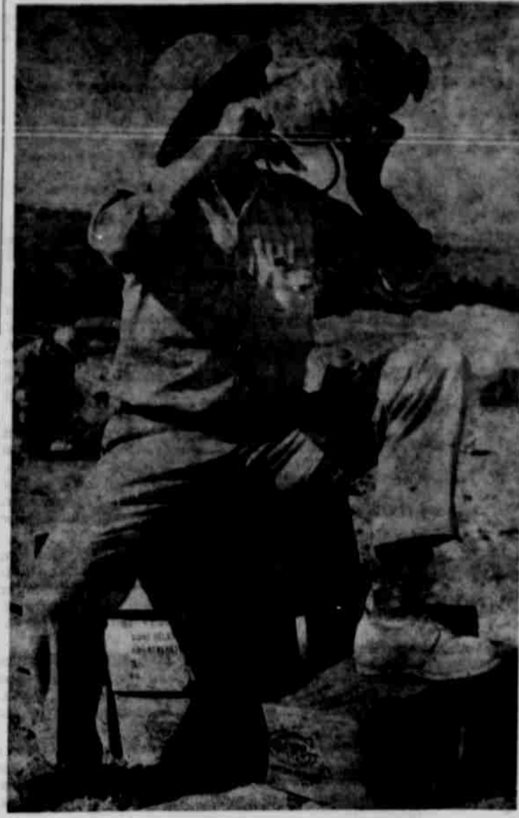
DYNAMITE AND SWEAT are the two major ingredients in current progress on Portland General Electric company's Round Butte dam on the Deschutes river as construction forces pioneer access roads into the 1,000-foot-deep canyon. PGE's thirsty Ernie Harmonson says a drink is a drink, but most agree there are better places to partake than on several hundred pounds of high explosives.
