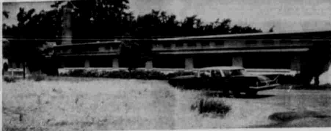
A. C. HOUGHTON School at Irrigon is one of the impressive buildings in that area and provides modern schooling for children there. (G-T Photo)
