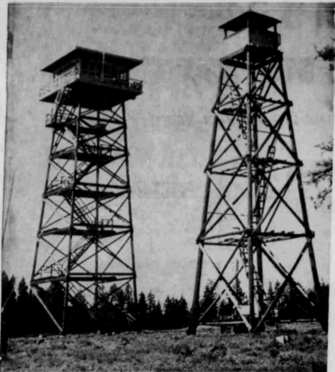
THE OLD and the new in lookouts are pictured in this U. S. Forest Service photo of the lookout towers at Wheeler Point. Although the towers are just out of the county, the rangers view forests in Morrow county from this point. The new tower at the left is a luxurious affair in comparison with the old structure.
