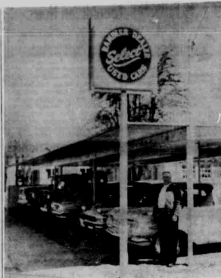
J. J. Farley Motor Co. has added a 6-car carport on its used car lot to better the facilities to serve the public. The new structure faces May street, at the corner of Chase. It is lighted so cars can be seen at night and a salesman is on call seven days a week.
