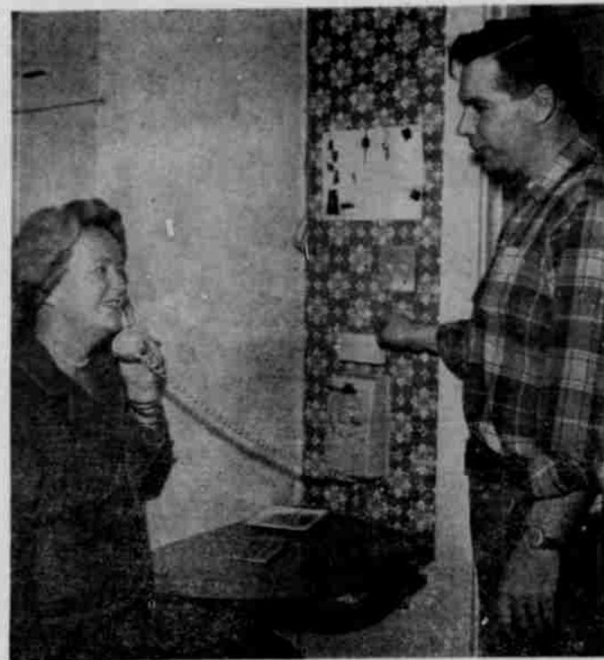
Mrs. R. Robert Smith, Portland, answers the front door from her kitchen using Oregon's first Home Interphone system which Dan Leahy, Pacific Telephone Northwest Installer, has just completed wiring in the Smith residence.
