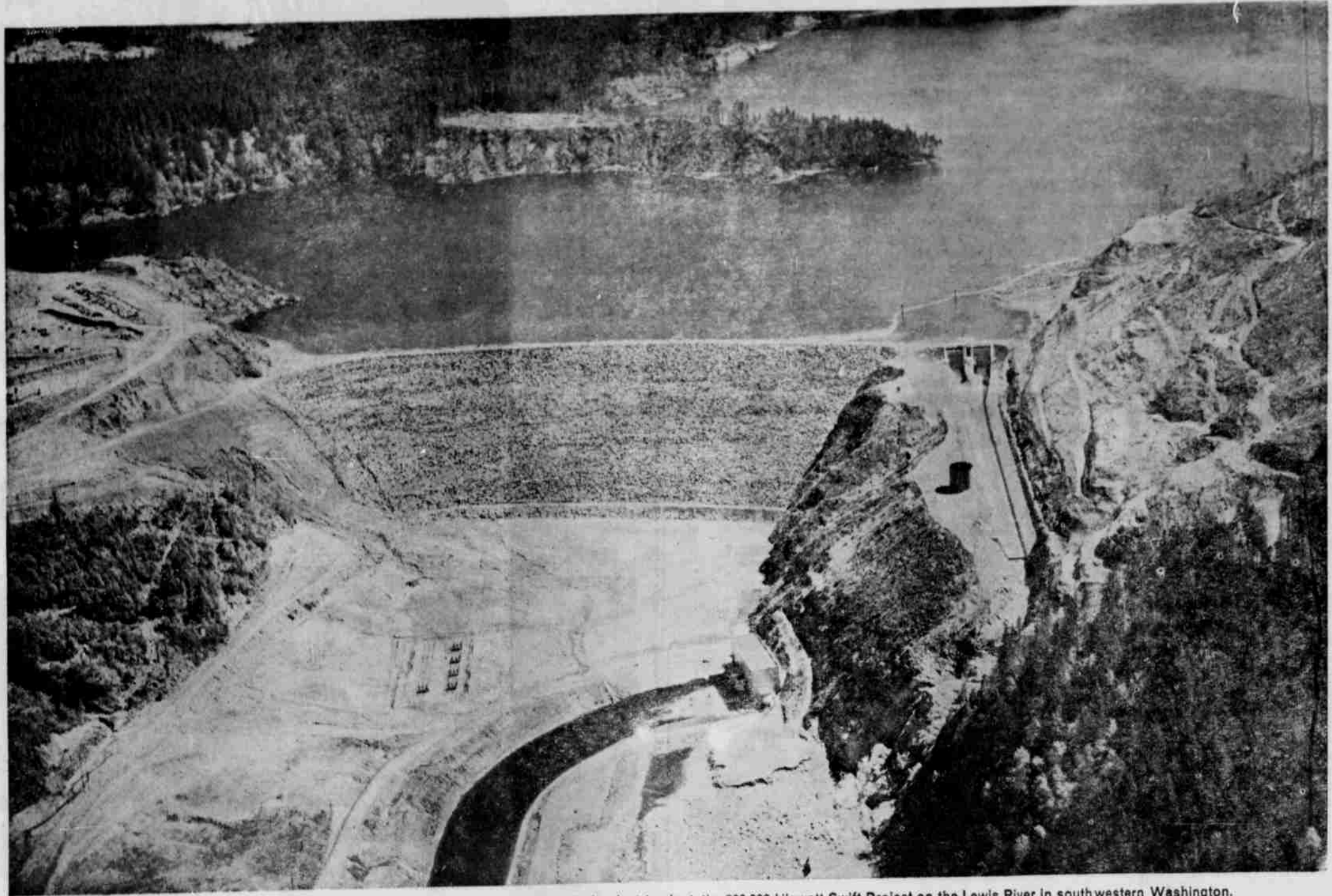
World's highest earth-fill dam is part of PP&L's newest and largest hydroelectric plant, the 268,000-kilowatt Swift Project on the Lewis River in southwestern Washington.
