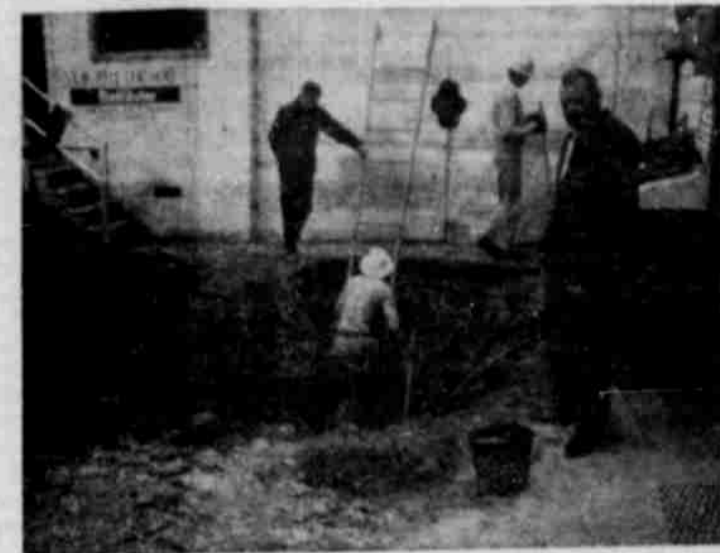
THE HOLE—here is one of several holes which have been dug during the past two weeks in an effort to find source of petroleum products which have been running into basement of Stefani's restaurant in Ione. When this picture was taken, hole was about 12 feet deep and bottom was saturated with gasoline. (GT Photo)
