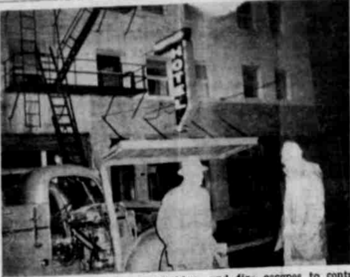
HOSE LINES were taken up ladders and fire escapes to control fire Sunday night which for a time threatened to destroy the 48 room Heppner Hotel. As windows were opened to air out the building, smoke poured from all sides.
