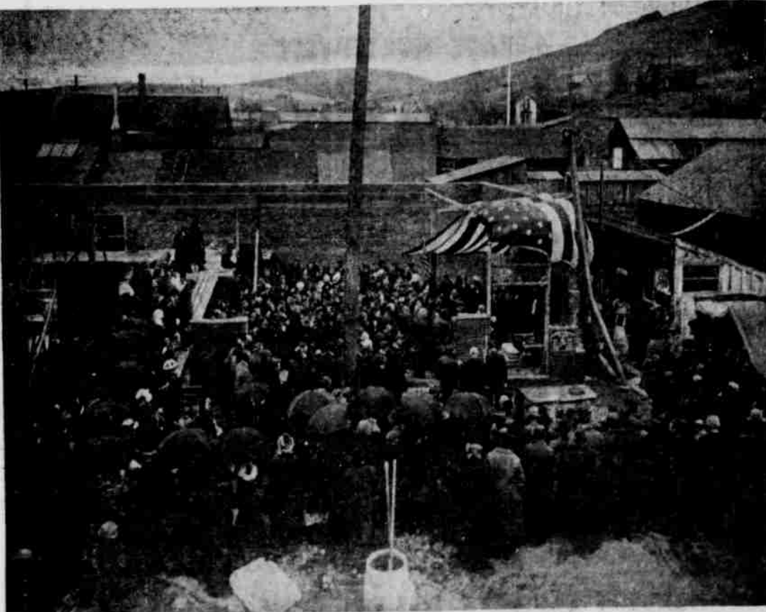
CORNERSTONE LAYING —A sizeable crowd gathered on a dreary, rainy day early in 1916 to witness the laying of the cornerstone for the new Heppner Masonic temple. This photograph was taken looking south and the camera was probably located on the roof of the building which now houses the Gazette-Times and the J J Nys law office. It is not known who the dignitaries are at the ceremony but it is obvious from the number of umbrellas that a good rain was coming down. This old photo is the property of Robert Lowe.
