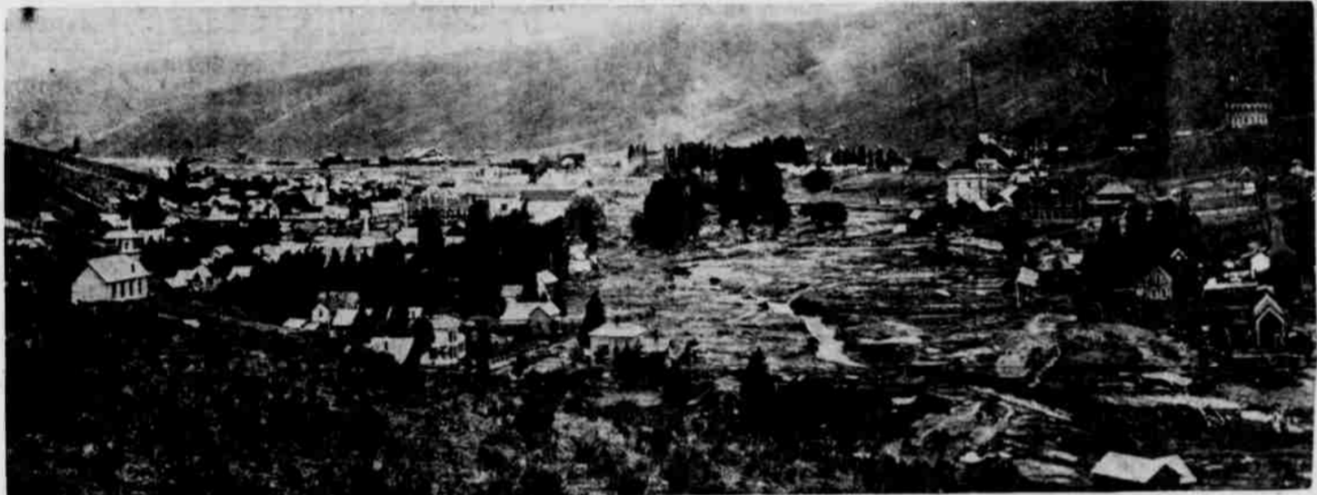
WHEN THE WATER HAD TAKEN ITS TOLL this was the way the south end of the town looked. This picture was taken from approximately the same position on cemetery hill as the above photo. It was in this upper section, where the valley is very narrow, that the water hit first. The torrent came into Heppner
