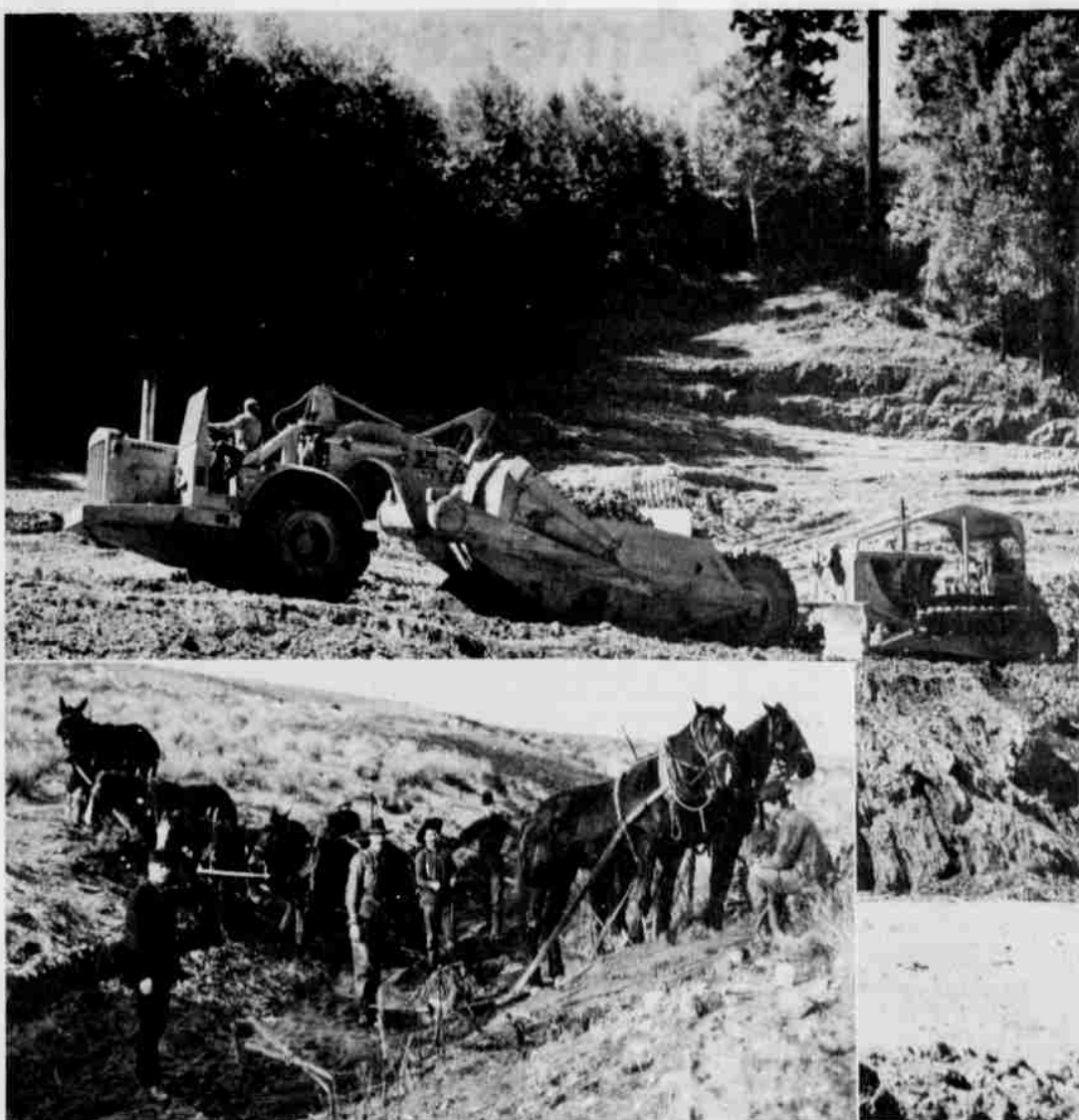
MOVING DIRT WAS TEDIOUS in early days. A man with a team moved 20 cubic yards of earth in a day. Now a tractor-scraper handles 800. Horsedrawn rig (inset) is digging an eastern Oregon irrigation canal (1900). The Caterpillar is building a Coast road.
