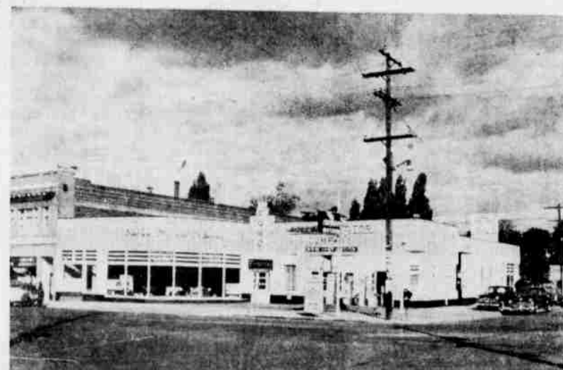
You'll be in good hands and you'll find up-to-the-minute service equipment... servicemen schooled in the latest factory recommended methods.
