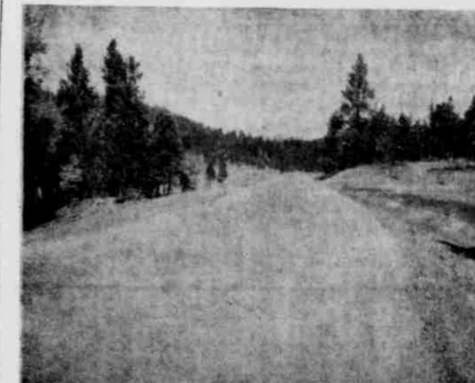
BIG IMPROVEMENT —Paving of nearly 4 1/2 miles of the Heppner-Spray highway over the mountains has recently been completed. This photo shows one of the new wide, smooth straight stretches which replaced the former narrow rough road. The new paving takes the improved road within about five miles of the summit. (GT Photo)
