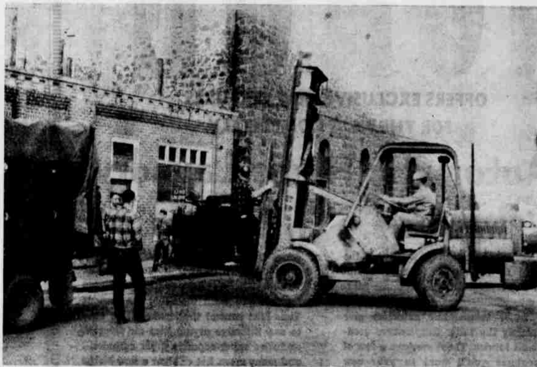
COMING IN—With the aid of a fork lift truck from Heppner Pine Mills, the GT's press, a 2-ton piece of equipment, is jockeyed through a front window of the plant. The press has a capacity of 3600 17 by 22 inch sheets per hour and its addition gives the Gazette-Times one of the most complete printing departments in this section of Oregon.
