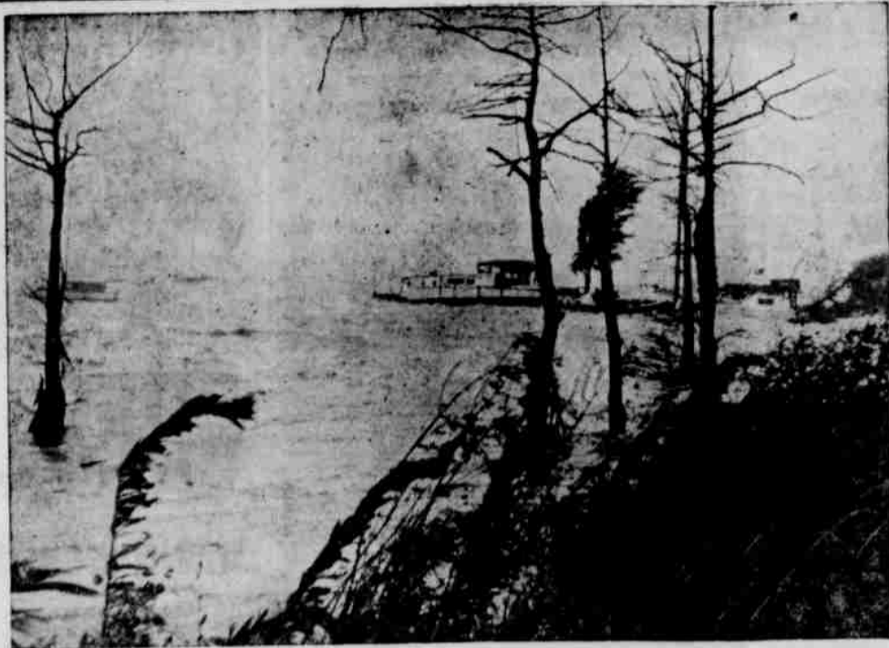
HIGH WINDS and waves herald the approach of Hurricane Audrey last June 27 along the Louisiana coastline near Cameron. Before the storm subsided, it had left at least 518 dead, 1,699 injured, and millions of dollars in property damage in one of the severest tests of State and local disaster organizations in the recent history of the nation. (Photo by Louis King, Lake Charles, La.)
