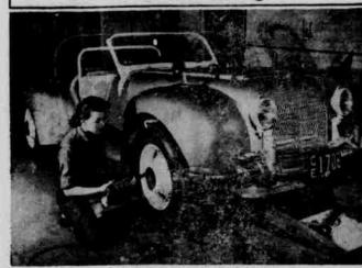
Grace Curry, Miss Autorama of 1956, checks her "Doodlebug" which she races Sundays down the drag strip at Woodbine, N. J. Capable of hitting 120 miles per hour, the car is a custom-made model, built by Grace herself. Here she checks over the wheel lugs for proper tightness with an Ingersoll-Rand Torque Control Impactool. First and only electric torque control wrench in the world with optional Torsion Bar Torque Control, the tool auto-
