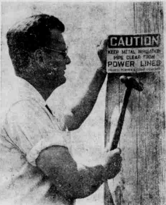
IRRIGATION SEASON SAFETY PLAN of Pacific Power & Light company includes renewal of posting "CAUTION" signs on rural area service poles near irrigation pumps similar to the sign being nailed to PP&L pole above. Sign reads: Keep Metal Irrigation Pipe Clear From Power Lines. Contact of up-ended sprinkler pipe with lines can result in serious shock.
