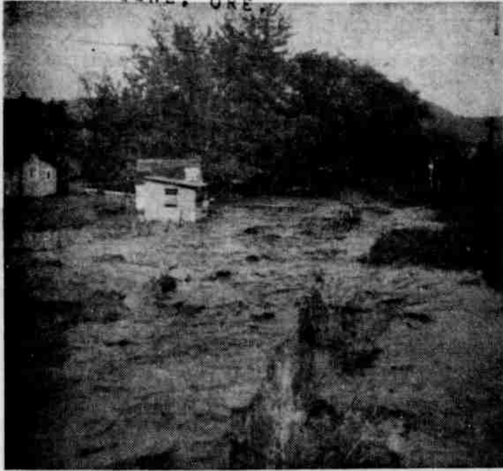
FLOOD AT ITS PEAK — Last Friday evening's flash flood was caught at its height by C. A. Ruggles as water was lapping at buildings in the extreme west end of town. This photo was taken from the Birch street bridge across Willow creek looking upstream. Little damage was done in town though youngsters had a field day after the water went down catching fish that had been stranded in puddles in fields. Thousands of fish were killed.
