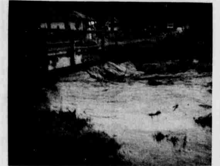
MUDDY DELUGE roars under the Alfalfa street bridge at the east city limits of Heppner. Before starting to recede the water raised at least another foot to put it well up on the bridge stringers which here were still above the surface. All city bridges and sewer line crossings withstood the water but water department crews had many anxious moments before the water started to drop.—(GT Photo)
