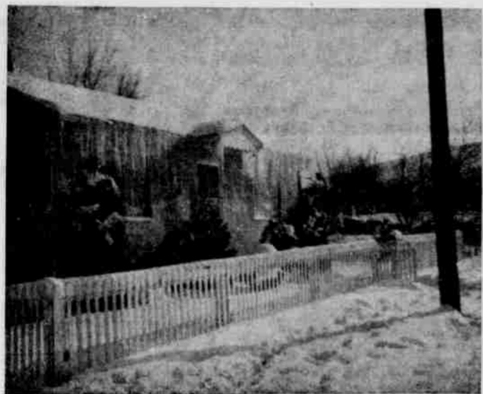
BEAUTIFUL BUT BOTHERSOME —Typical of most houses and buildings in Heppner during the past two weeks is this array of icicles hanging from the eaves of this home on South Court street belonging to Alta Cutsforth. Many buildings were having troubles with icicles weighing down eaves and freezing under shingles, pushing them up. Continuing sub-zero temperatures have only added to the length of the icicles as some thawing occurs during the day. (GT Photo)
