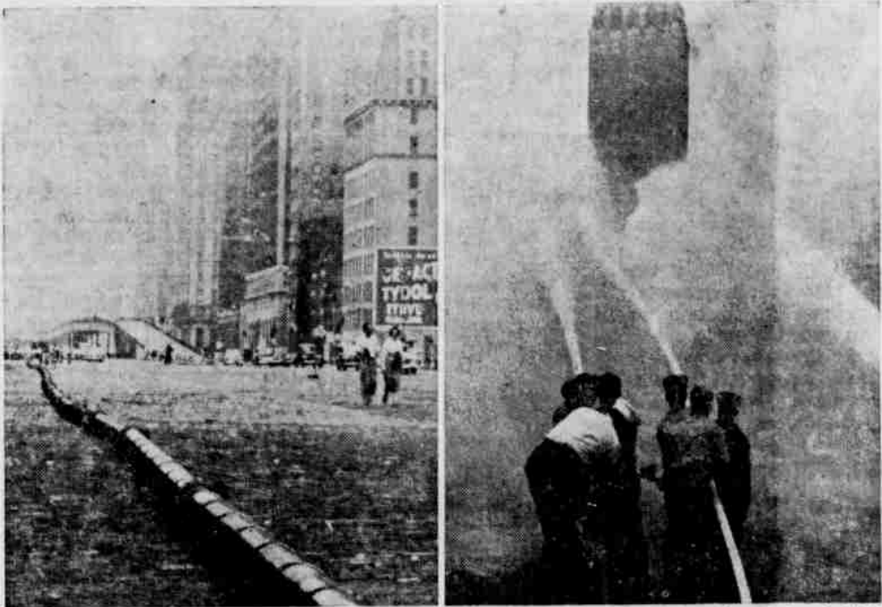
DEMONSTRATION OF PIPE in New York City which can be laid quickly over rough terrain to carry water for fire fighting, city water supply or to pump out flooded areas. This flexible coupled pipe is stored by the Federal Civil Defense Administration in warehouses throughout the nation for use in emergencies. New couplings allow pipe to be laid without leveling it.
