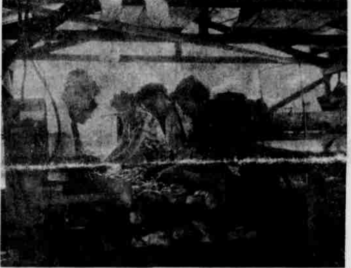
POTATO GRADING is shown closeup. The number one washed potatoes move on a conveyor into the foreground where they are sacked. Number two spuds are shunted off into another conveyor between first two girls on the right and the culls are kicked off into another conveyor to drop into a waiting truck to be hauled off. About 80 percent of all potatoes handled here are graded number ones.
