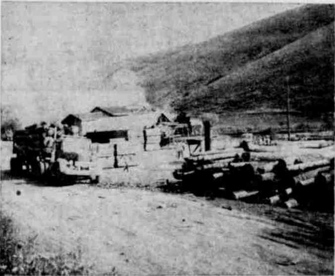
A LOAD OF LOGS, is being dumped and will be stacked in the cold deck, a small part of which is shown in the right foreground. The main mill in the background got into limited operation last week, but it is expected that it will take some time yet to work all the bugs out of the operation. The plant cuts only 2x4's 8 feet in length.
