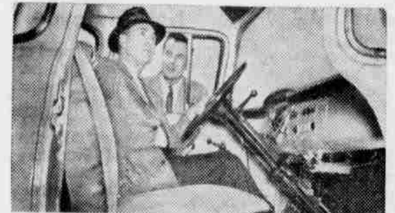
Modern cabs with High-Level ventilation, panoramic windshield and concealed Safety Steps.
